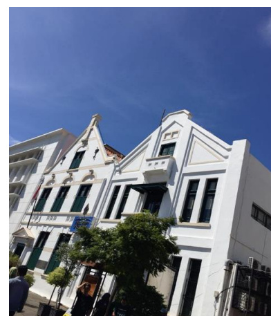
Figure 4 Kota Tua Jakarta: some Buildings that have been Adapted with New Function as Museums
